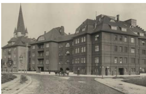
tenement houses in Sztabowa Street – the second decade of the 20th century and tenement houses in Sztabowa Street today
